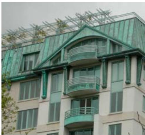
Copper roofs and flashing are fabricated into standard or custom shapes by a number of manufacturers. Roof panels (see photo at left) are commonly from 0.4 to 1.0 m (16 to 36 in) wide, and up to 3.1 m (10 ft) long, with other sizes available via special order.
