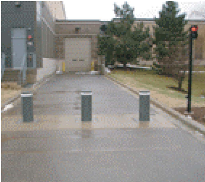
Exhibit 5-6. Delivery restriction bollards.
